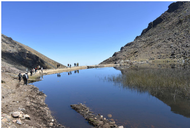
FIGURE 5 | The dam of Weetacocha rehabilitated (July 2025).
