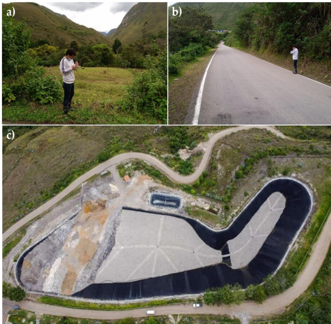
Figure 5. Field validation. a) and b) Visual inspection of potential areas. c) Inspection of the current landfill
